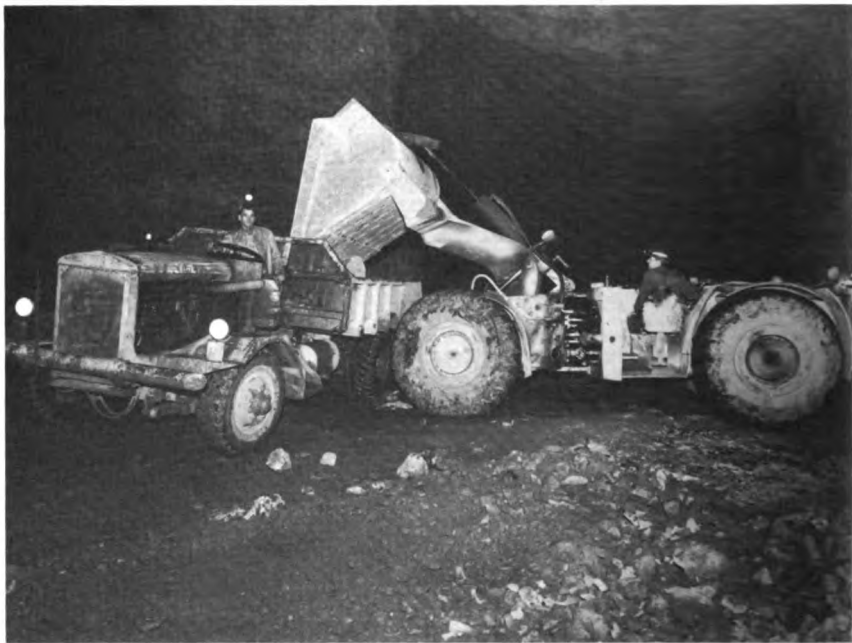
FIGURE 11 Diesel powered underground loading and haulage units.
